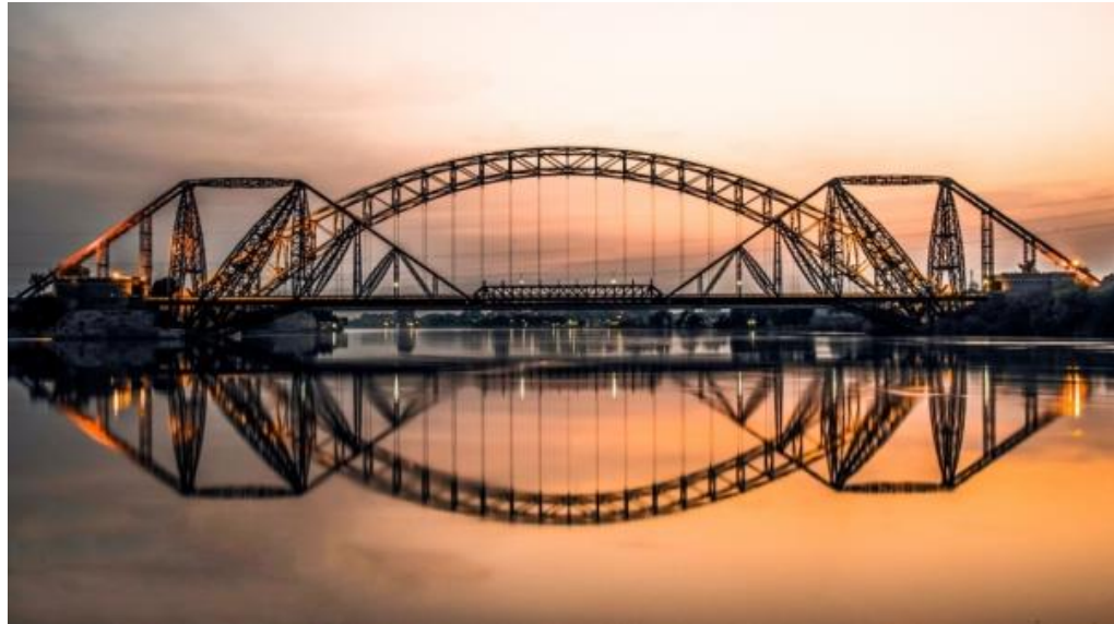
Lansdowne Bridge (Cantilever Bridge) Sukkur
